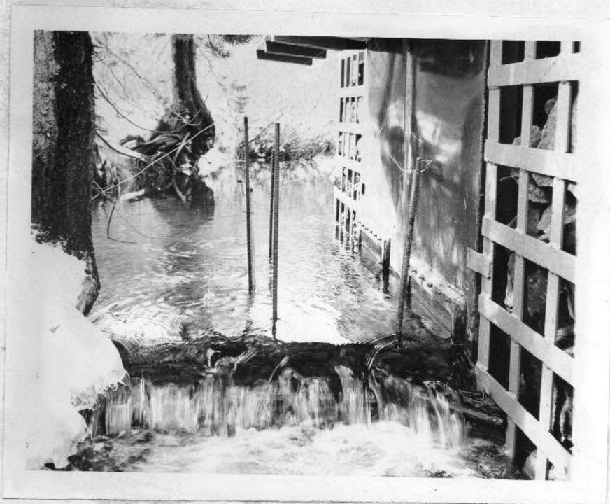
Thermocouple Stations on south side of tank, used in the study of ice formation and dispersal and its concomitant effects on fish life.
