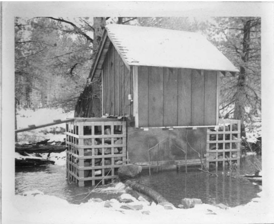
Underwater Observation Tank as used in the winter of 1953-54. The wires leading from thermocouple stations placed at various positions in the stream bed, are seen just below the middle section of the top of the tank. Rock racks at each end counteract buoyancy.
